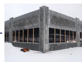
The Lifeworks Medical Office Building was built to offer the maximum amount of medical facility space within the design footprint. The precast concrete walls have a number of unique features cast into the exterior face of the panels to add depth and interest to the structure.
